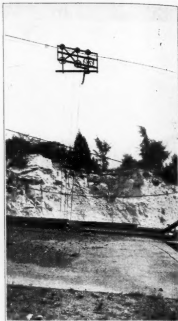
Carriage with Dumping Controlled from Hoist House
